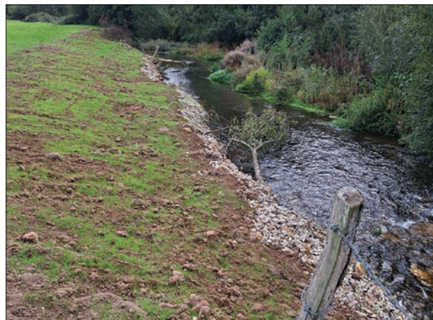
Riverbank after restoration
