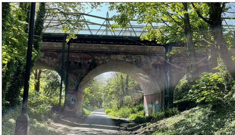
The three arch bridge supporting Buxton Road
