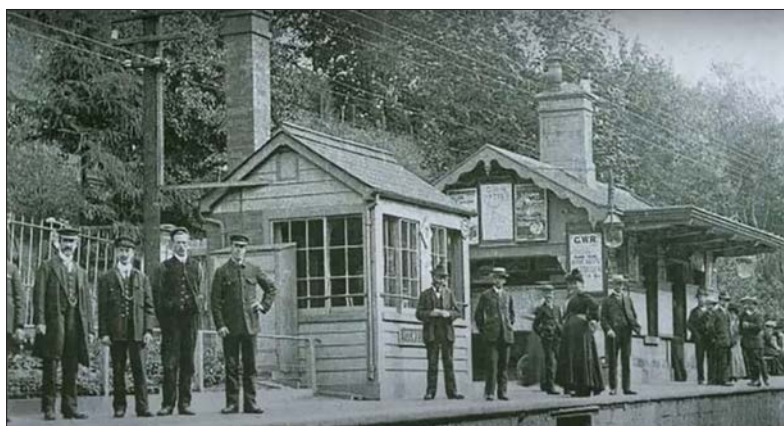
Above: Rodwell Station and Below: Loading stone onto railway trucks at Priory Corner
